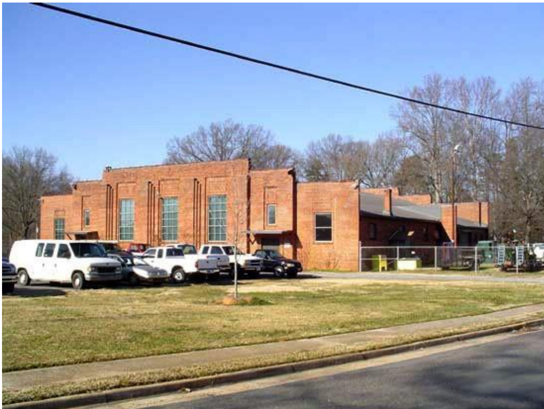
Fort Mill Armory. ca 1938. Image property of SC Department of Archives and History.
